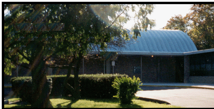
FORT ISLAND PRIMARY SCHOOL
